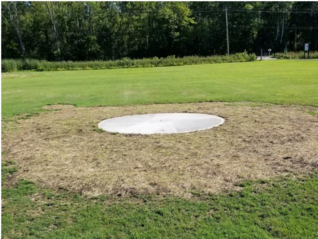
Here's the UCC pilot's pad after the ground-scaping was completed:
